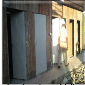
local workers ablution block
