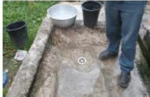
Waste water piped to normal drainage system for NBPOL
