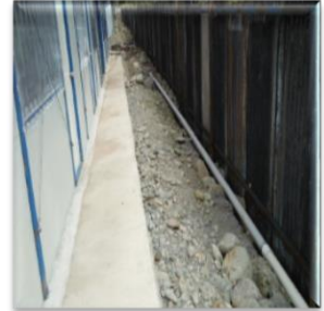
Drainage at the back of living quarters 2
