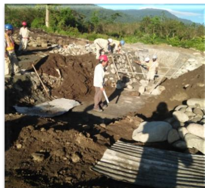
Workmen working on diversion channel
