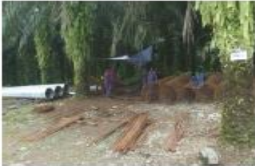
Workers at work at what is supposed to be a workshop
