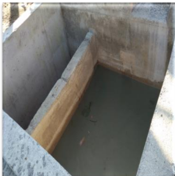
Access water drainage
