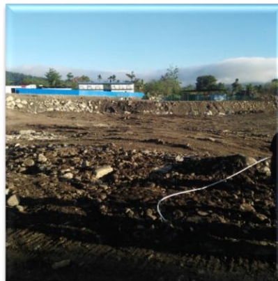
cleared site for powerhouse
