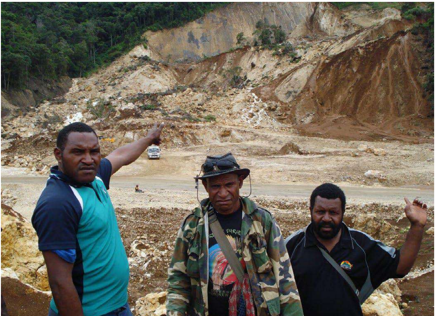
Tumbi landslide near Exxon-Mobil gas operations © LNGWatch/PNGblogspot.com
