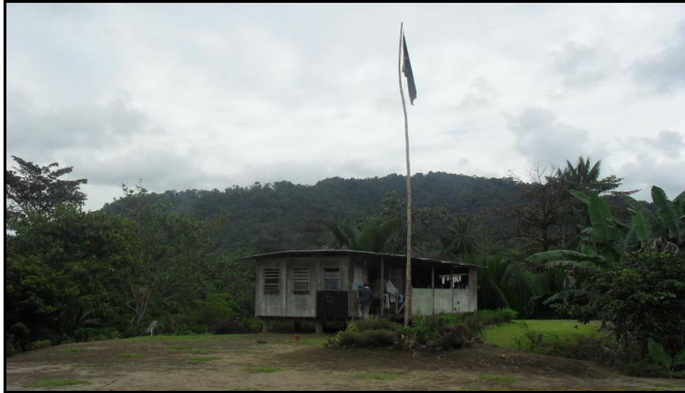
Figure 30: Grade 5 classroom at Wabo Primary School (built by InterOil in 2001)
