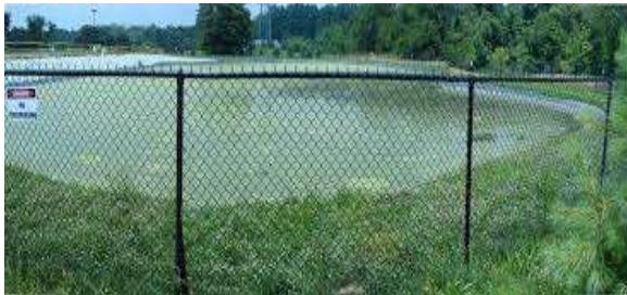
Sewage holding ponds (Photo by Water PNG)
