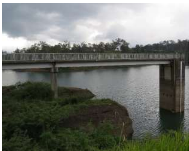
Sirunumu hydro dam in Sogeri, Central province (Photo by E. Kaitokai)
