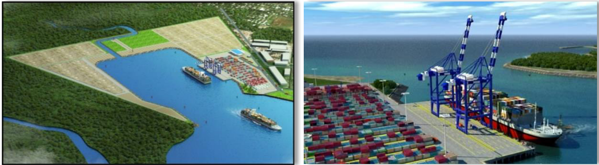
Figure 2-1 Tidal Basin Phase 1, Wharf and Berthing Facilities, Cranes and Container Storage
