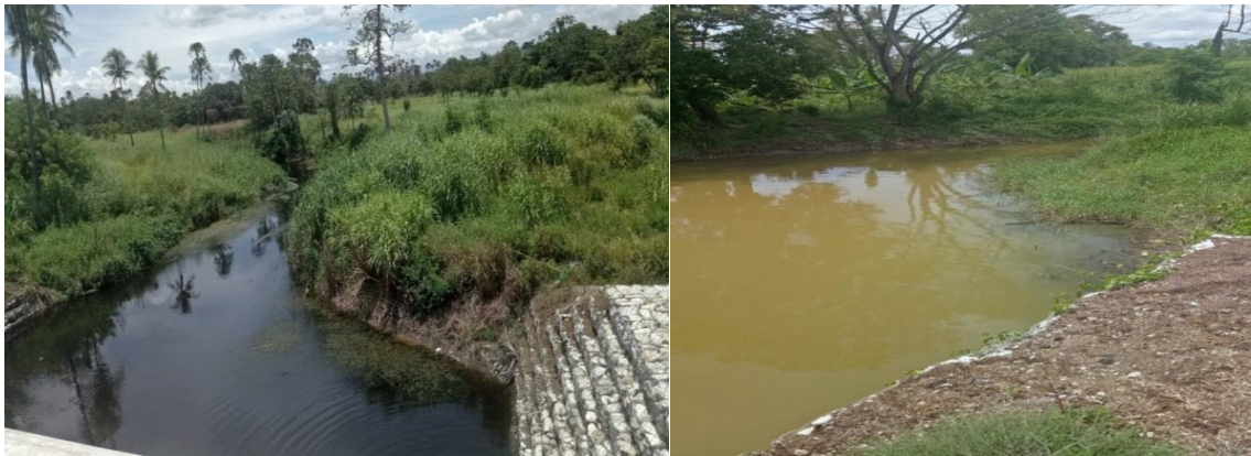
Photo 3 & 4 Stagnant Water at Sivitatana Site and Kokebagu
