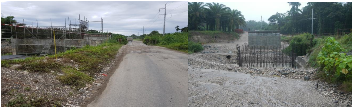
Photo 7 & 8: A Site Remains Closed and Secured during Work Suspension
