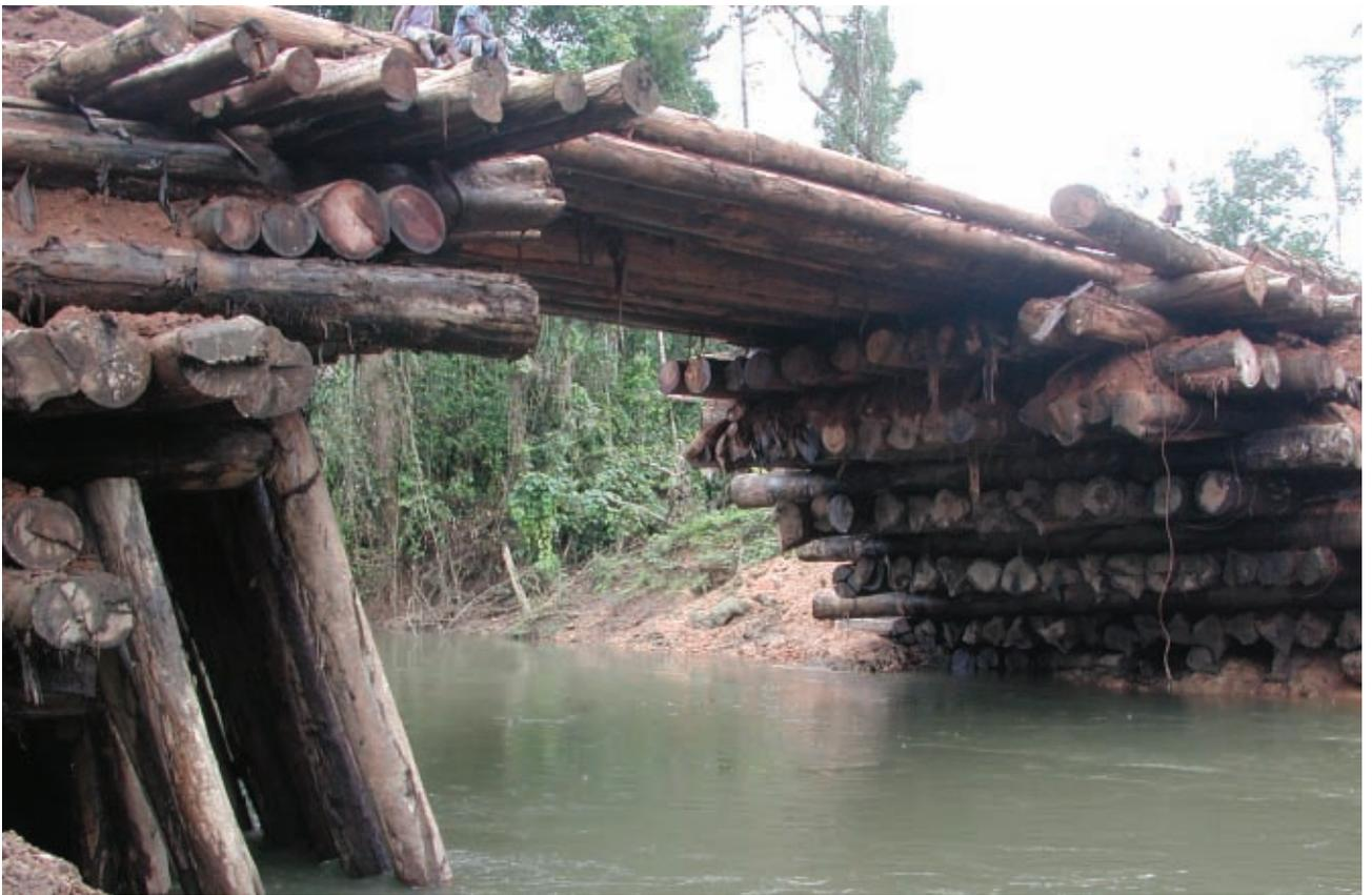
Plate 7: Large numbers of trees are used in the building of temporary bridges. Here approximately 250 trees are in the construction of this bridge in central Wawoi Guavi, Western Province. In this concession, several bridges of this size are constructed within each kilometre of roading.
