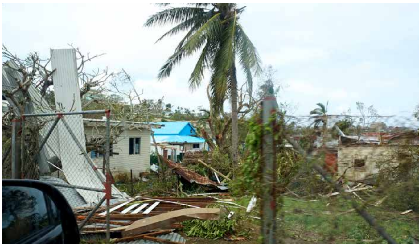
Natural disasters such as cyclones, floods and tsunamis generate large quantities of solid and liquid wastes, which can pose risks to public health. Photo: C.Siota/SPREP
