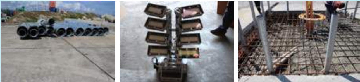
Upgrading lighting to reduce energy consumption at Honiara Port
