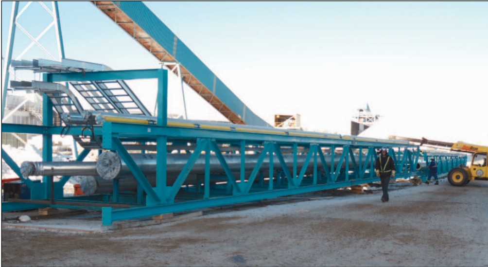
Plate 7.8 – Pipe Bridge Modules (Piping Pre-tested, Insulation Installed, Cable Trays Loaded)
