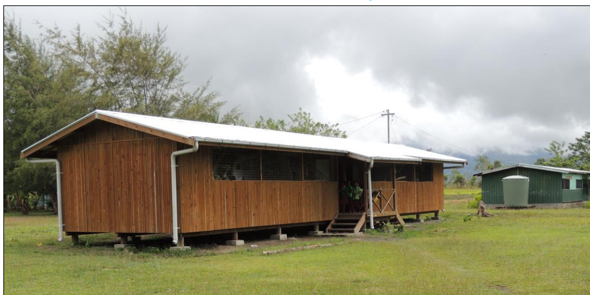
Plate 6.37 – Tararan Elementary School
