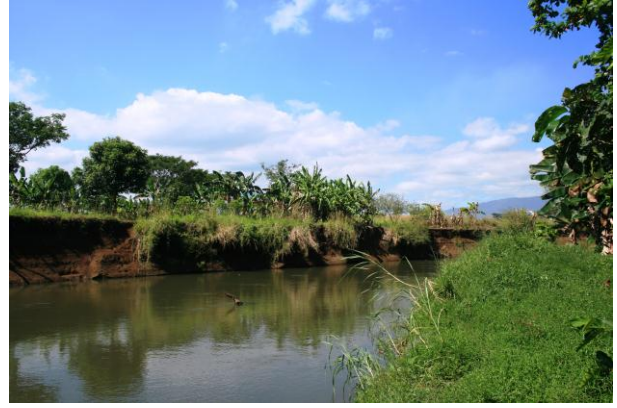
Photo 5: Visible effects of erosion of the Laloki River
