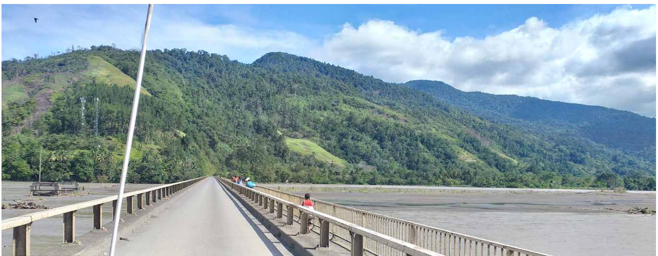
The Markham Bridge outside Lae on the Wau-Bulolo Highway, Morobe Province, a key economic zone with forestry, mining and agriculture developments. (Biatas Bito)
