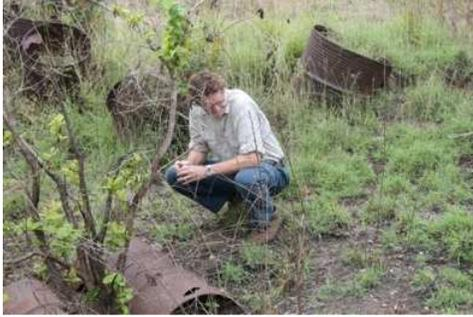
**Figure 32 AA Site close up of corroded fuel cans used as reinforcements – note holes**
