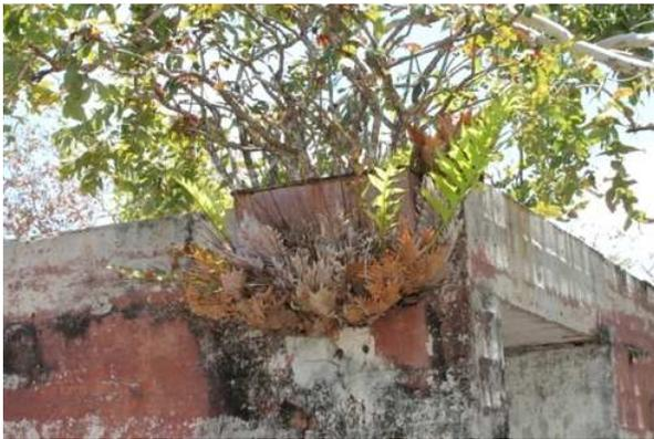
**Figure 24** Plant damage to building
