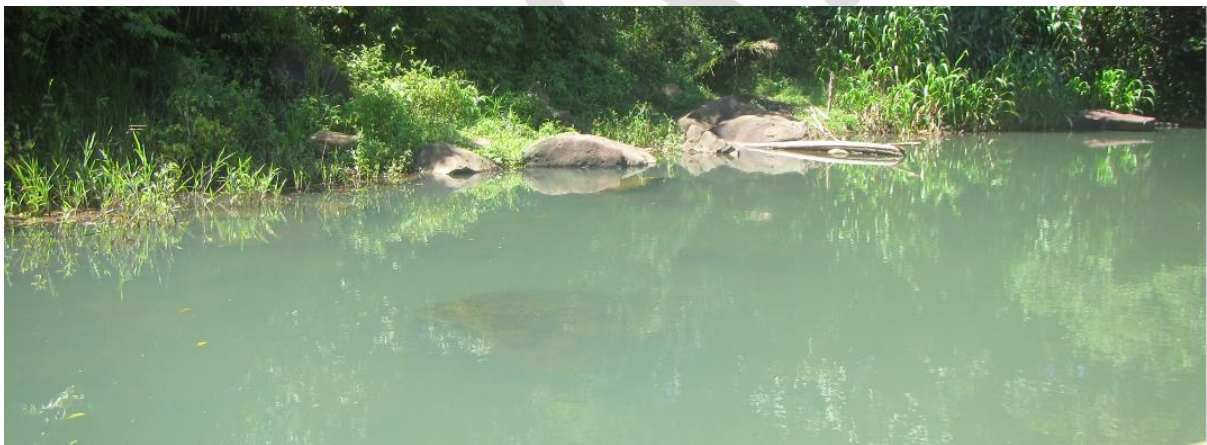
Figure 45. Upstream of Sirinumu Dam (April 2018)
